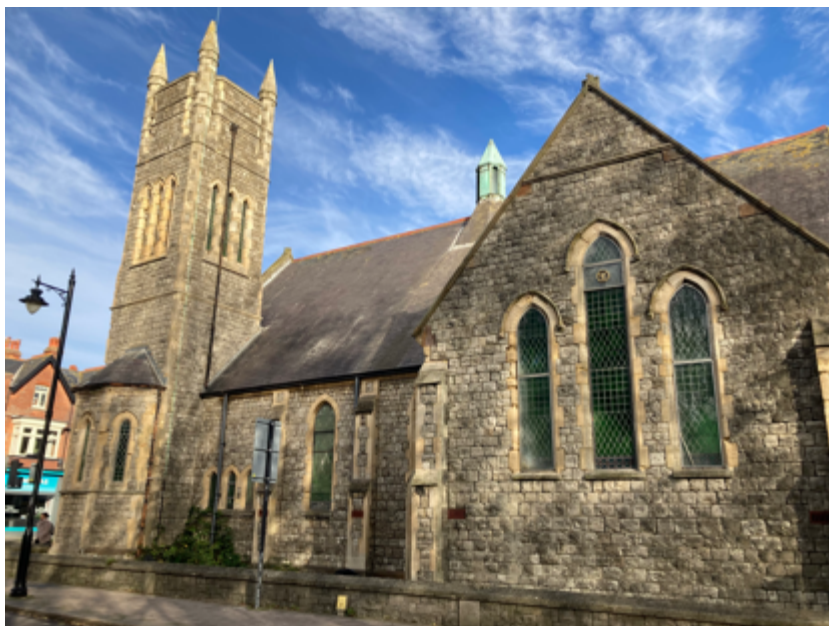
Figure 30: Former church of St James
