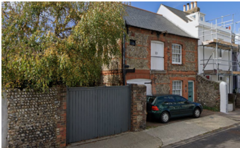
Figure 48: Park Road, west side
