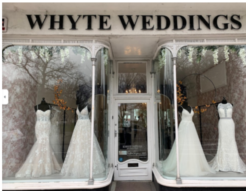
Figure 23: Shopfront at No.6 The Broadway
