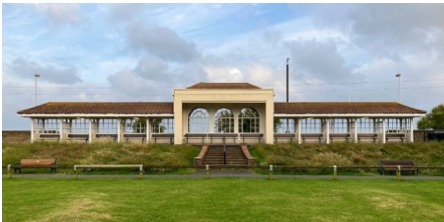
Figure 44: Shelter at southern end of Denton Gardens
