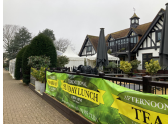
Figure 62: Poorly sited services and temporary installations
