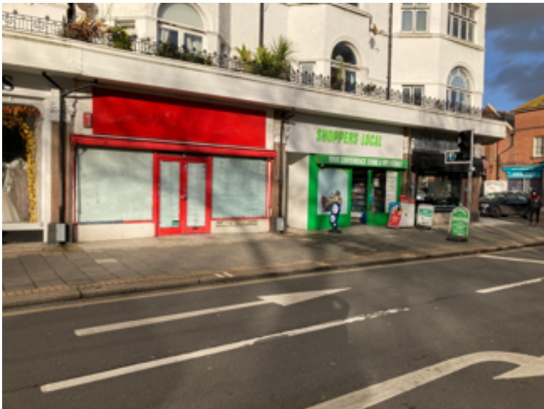
Figure 61: Poor quality shop fronts along Brighton Road
